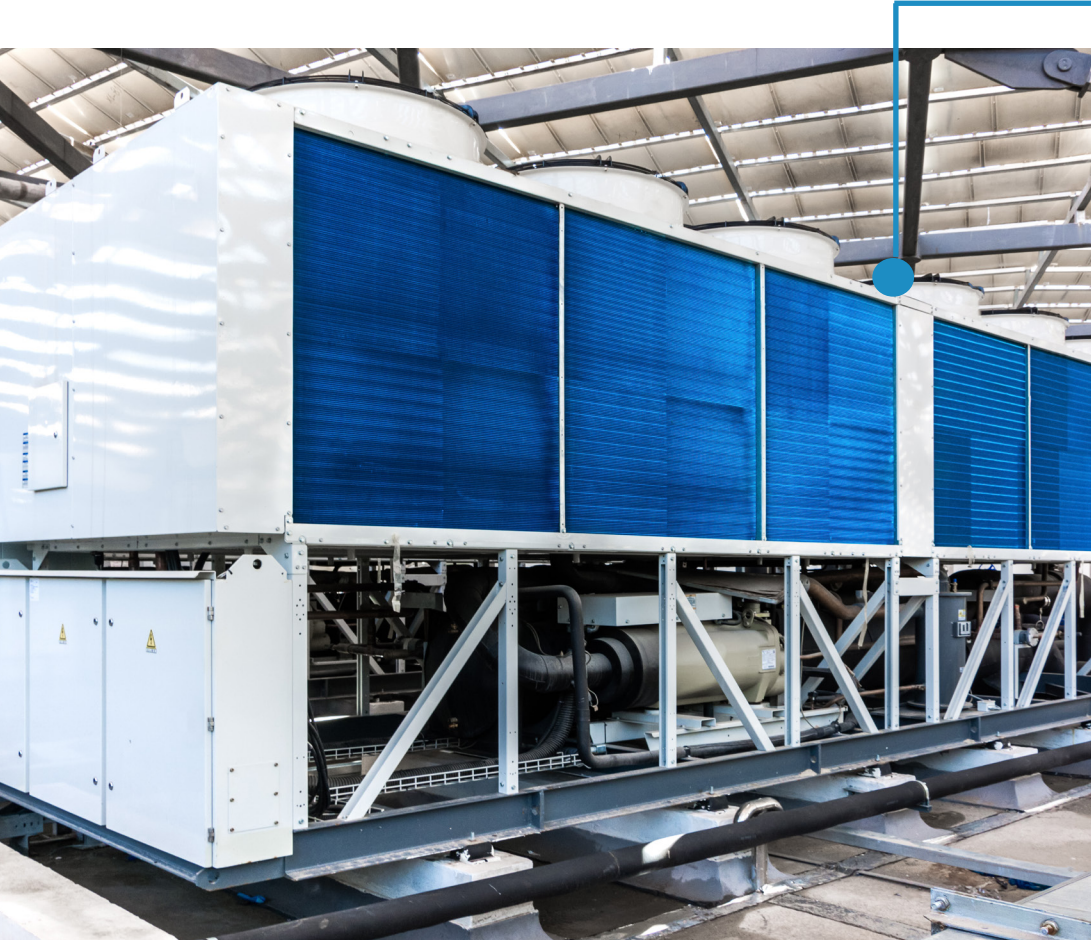
Heat pump system of big distribution warehouse
